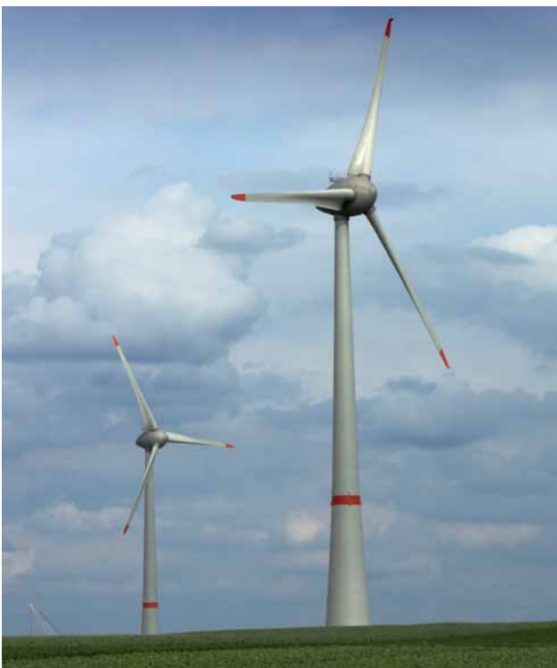
Enercon E-126 Turbines in Belgium. SOURCE: STEENKI
