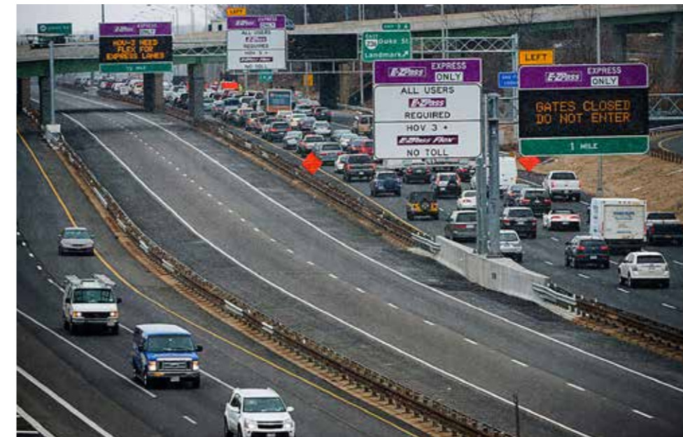
HOT traffic lanes / express lanes in Virginia using a 29-mile portion of existing reversible lanes
