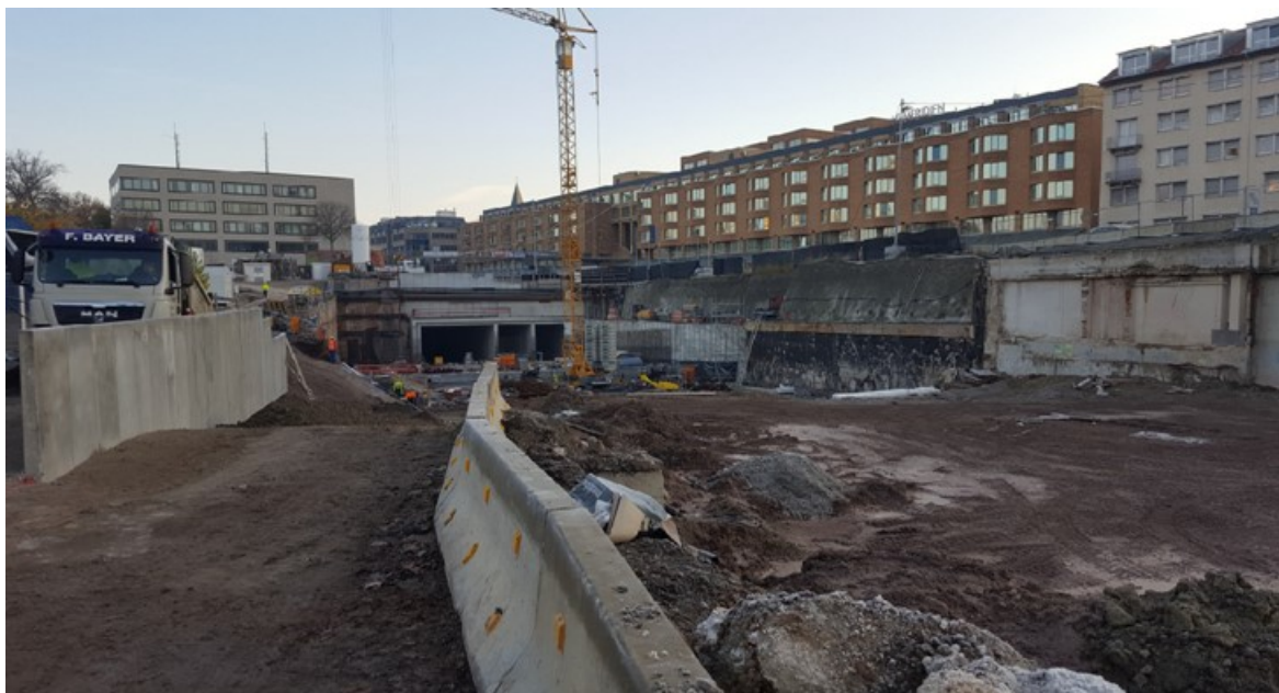
Picture 2 - Construction works on the Stuttgart 21 station
