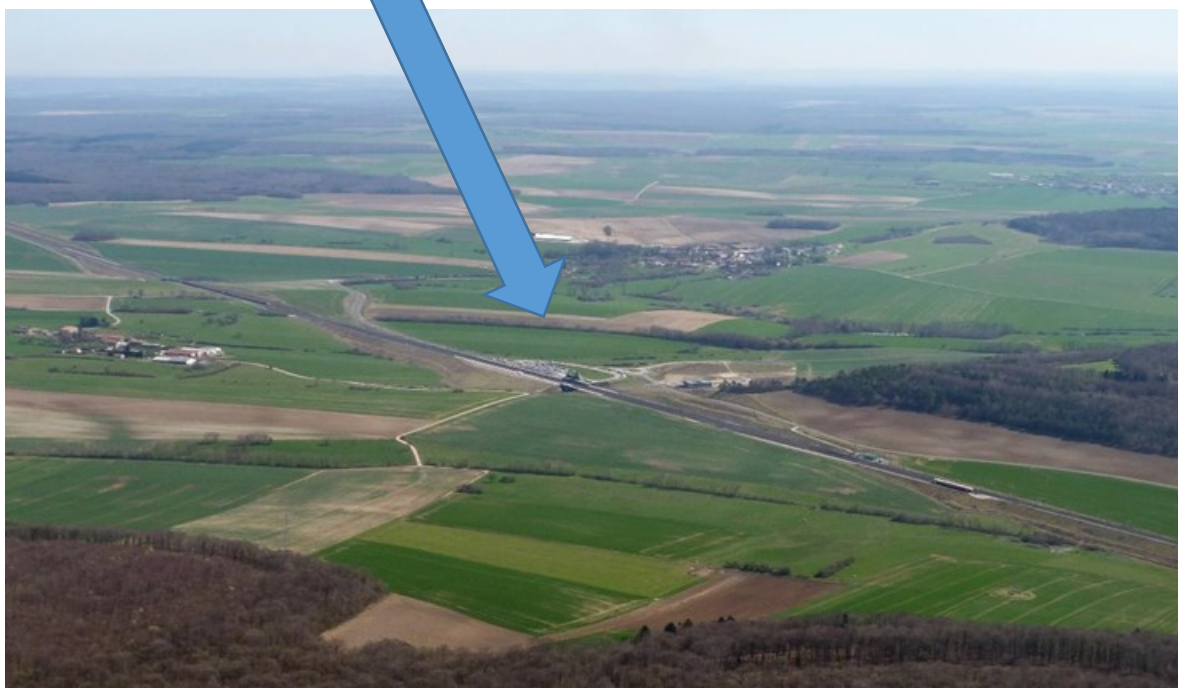
Picture 3 - The Meuse TGV station
