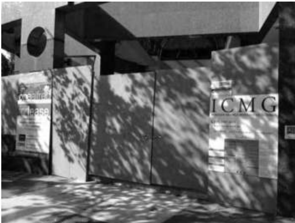
Figure 4-11: Temporary George Street Driveway at Goldfields House
