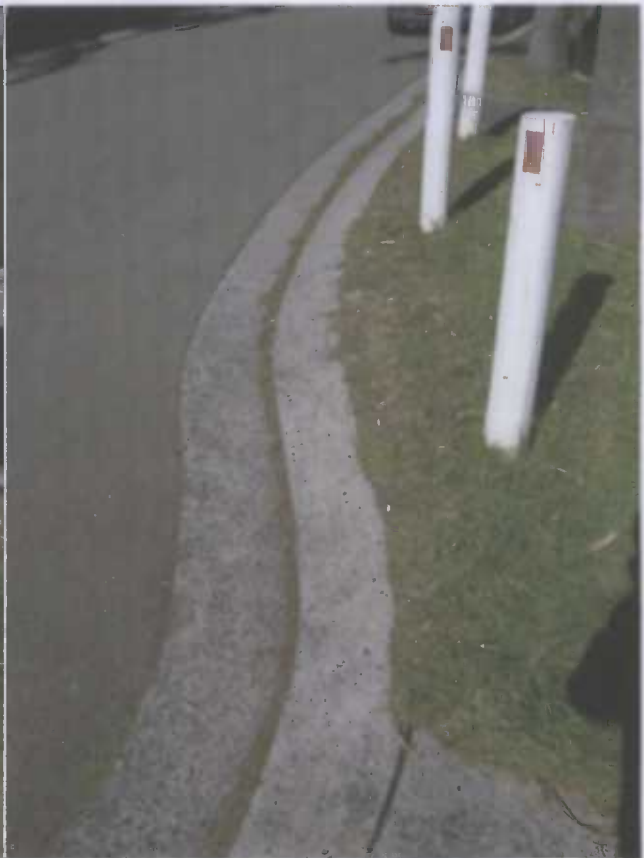
Photograph (8) Lodge Lane Street Kerb (Kerb Detail Next To Road Crossing)
