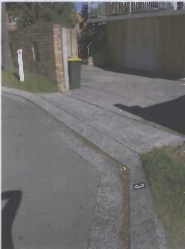
Photograph (7) Lodge Lane Street Kerb (Kerb Detail Next To Road Crossing)
