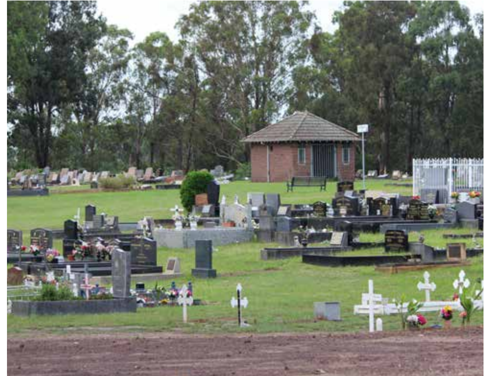
View to former Diggers Shelter from the north
