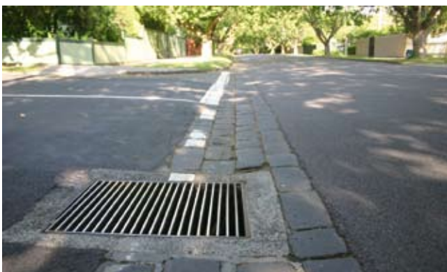
Figure 1 – Drainage grates with bars parallel to the direction of travel pose a serious risk to cyclists
